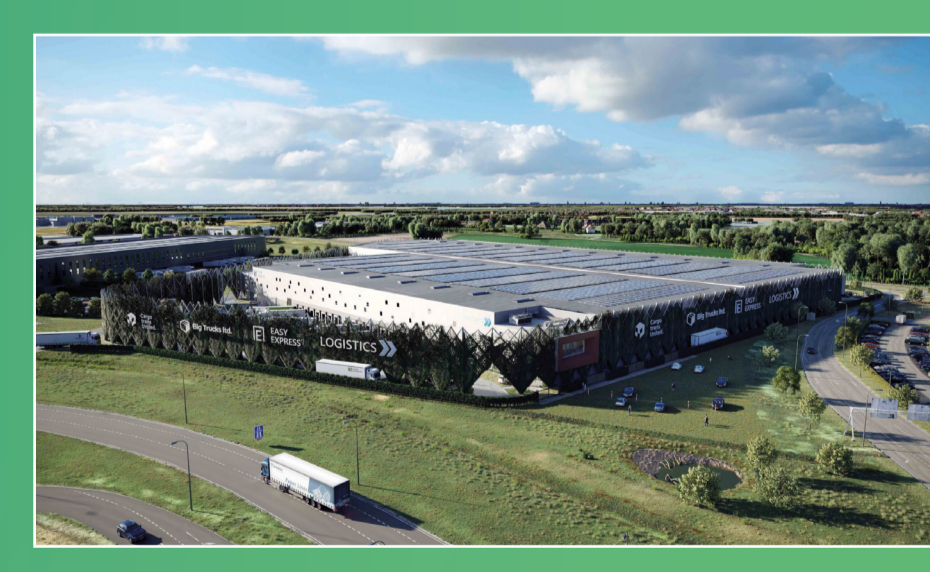
Ara Almelo Almelo (Twente) Stellar Development/Heembouw
